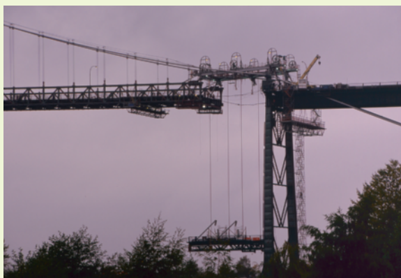
Exhibit 3—Raising panel 1, daybreak, September 9, 2000; photo from the former project website, © 2000 Stuart McCall/North Light.
